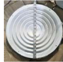
SAD (Round) Supply Air Diffuser
